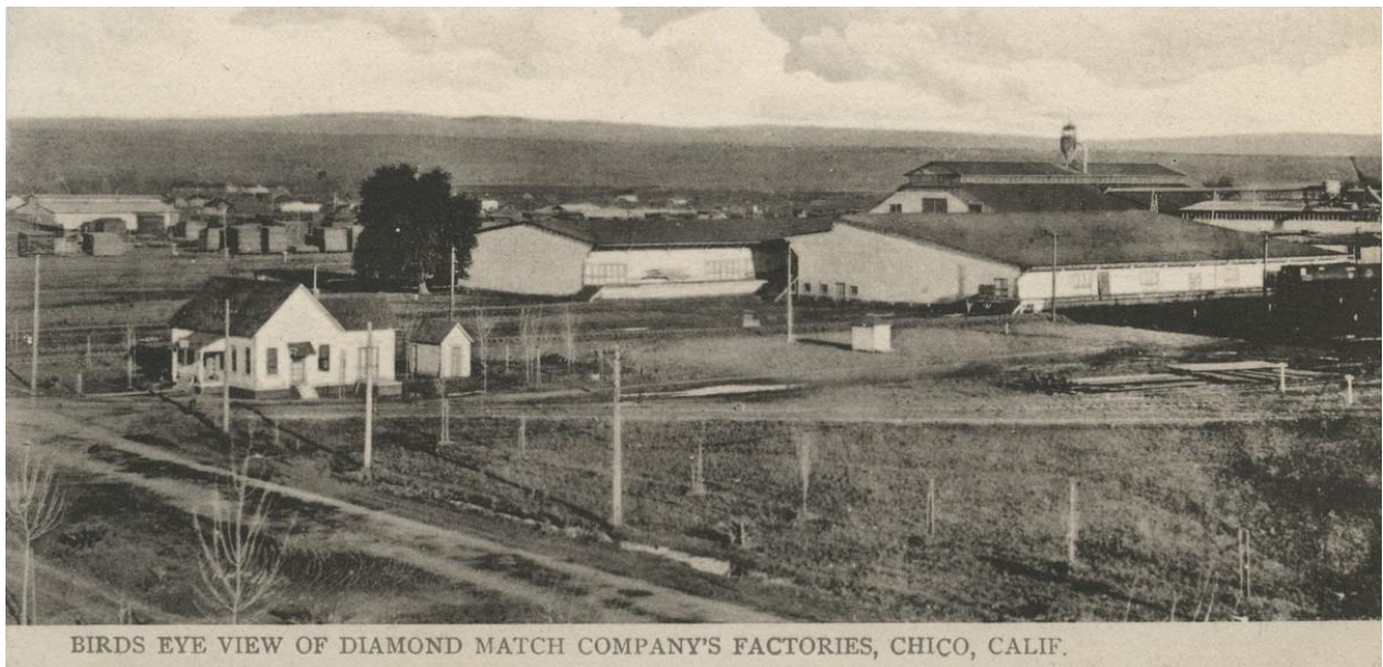
This shows a circa 1906 photograph of the site.
