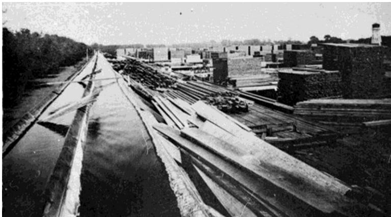
A view of Sierra Lumber Company Flume located between East Eighth Street and Humboldt Road east of Pine Street in Chico in 1907.
