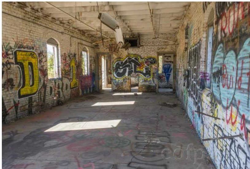
Inside View of the small storage building
