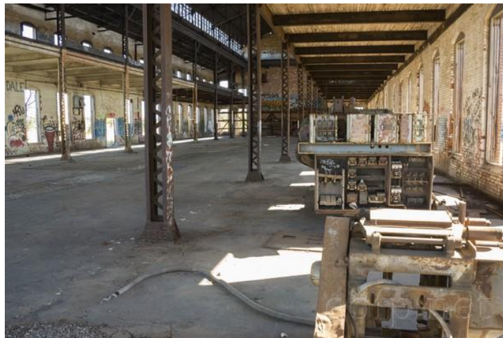
Inside view of the Engineering Building
