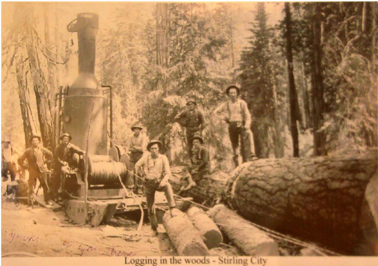
Steam powered "donkey" winch with a "line horse."
