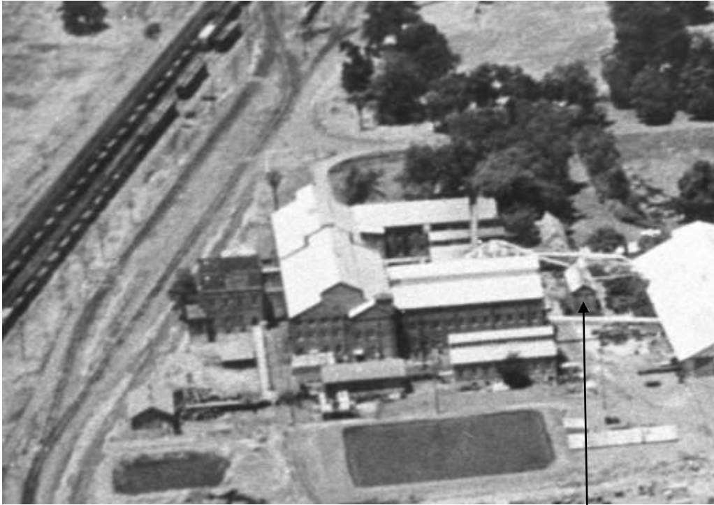
1965 view clearly showing the Small Storage Building
